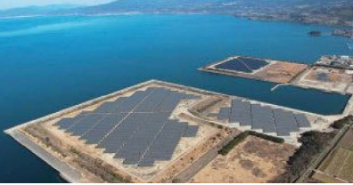
Omura Mega Solar Power Plant
