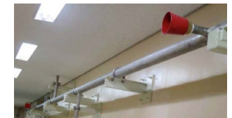
Automatic fire extinguishing system (Halon fire extinguishing system)
