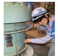
Checking for abnormal sounds with a stethoscope
