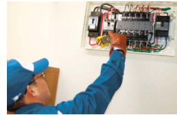
Distribution board inspection
