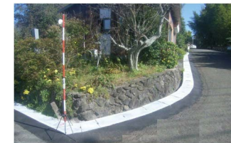
Support for improvement of access roads, etc. (installation of gutter covers)
