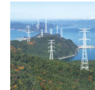
Power transmission towers
