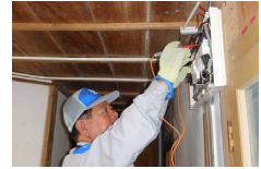
Indoor wiring inspection (Kumage Distribution Office)
