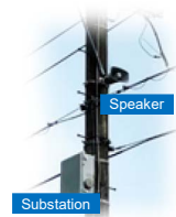
Installation on utility poles
